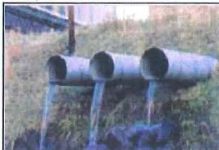
*An outfall that is sending water into a storm drain or stream when there has been no rain in the last 72 hours.*
